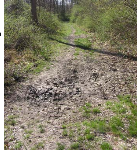
Trail widening has occurred where trail users have tried to avoid muddy places in the trail. When using trails hike or bike through muddy areas to prevent widening of the trail.
