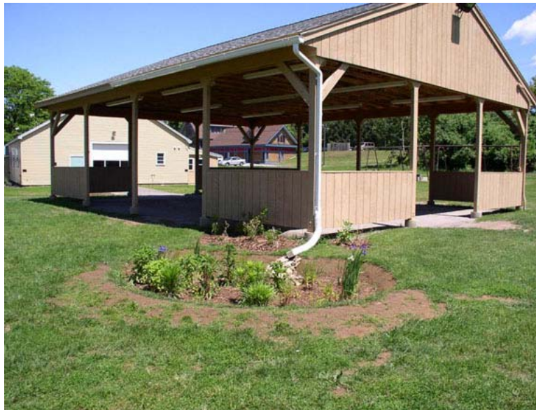
Image Credit: A newly installed Rain Garden http://www.ct.nrcs.usda.gov/rain-garden_tac.html
